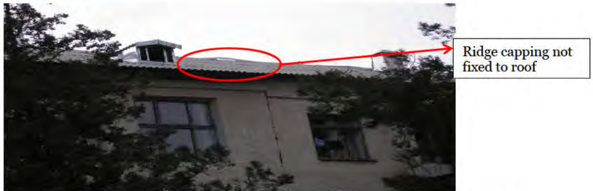
Fig. 30 - Poor quality roof renovation
